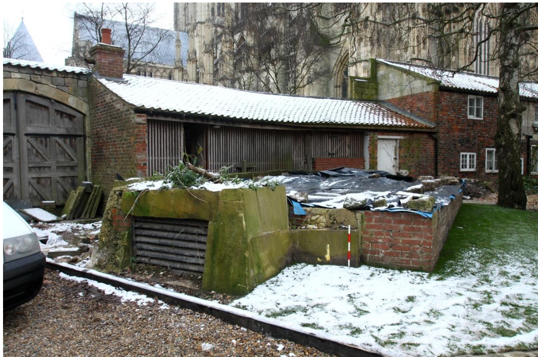
Plate 1 View of the generator enclosure and potting shed, looking SE
