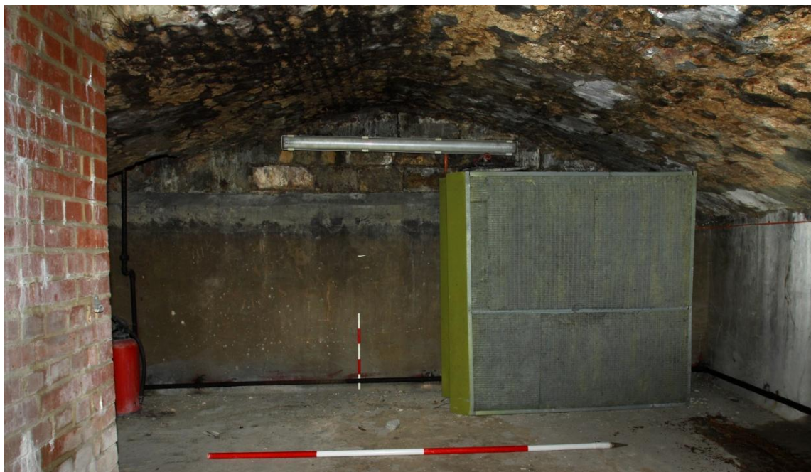
Plate 4 View of interior of the cellar, looking SSW. Note the concrete lining to the cellar walls excepting the uppermost part at end.
