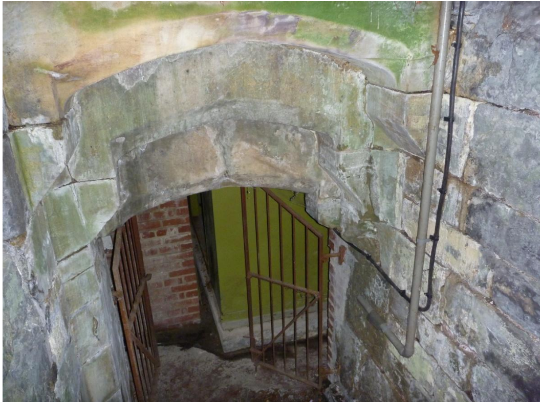
Plate 6 Entrance to the cellar and generator enclosure, looking WSW
