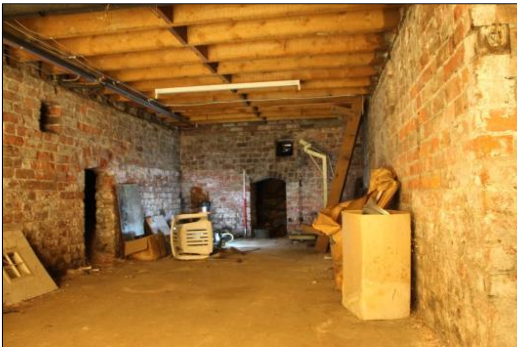
Plate 30: Room B1, looking southwest
