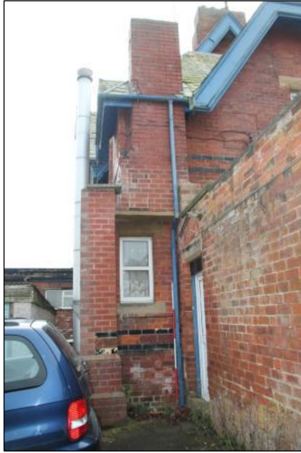
Plate 25: North corner of the cottage
