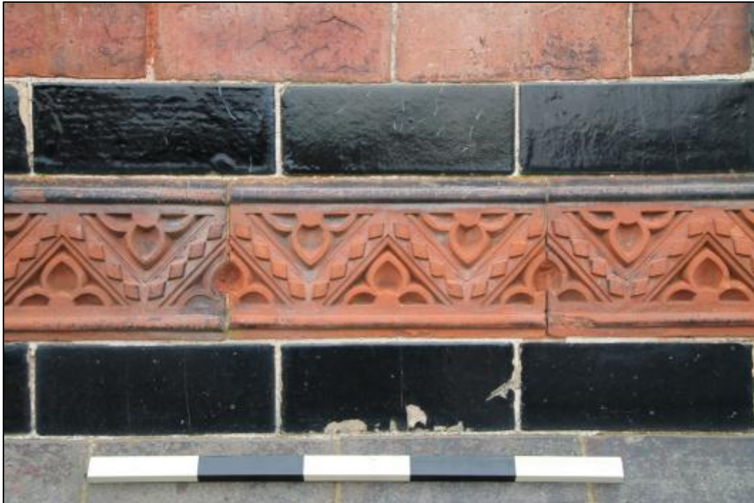
Plate 3: Detail of terracotta moulding forming band around structure
