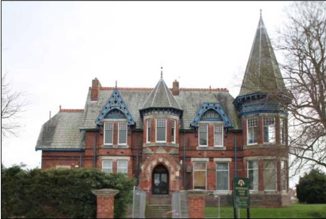
Plate 1: Southwest elevation of Burnholme house
