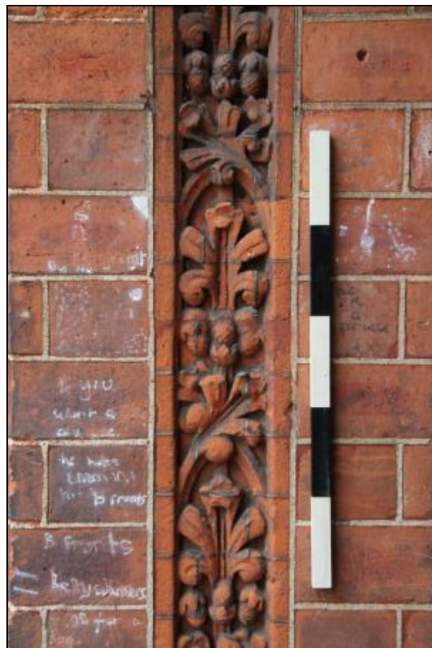
Plate 4: Detail of terracotta moulding around intrados of porch arch
