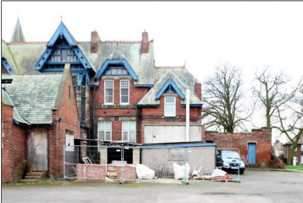
Plate 17: Northern bay of northeast elevation of main house and cottage
