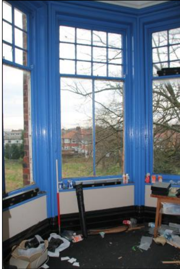
Plate 82: Room F2a, looking southeast
