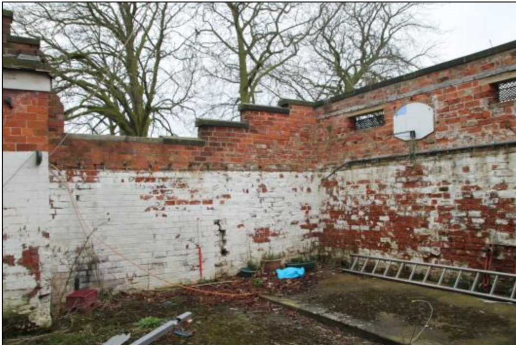
Plate 26: General view of enclosed yard, looking west
