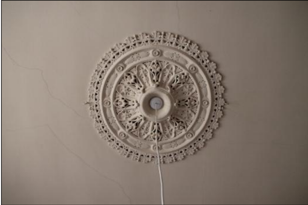
Plate 90: Detail of ceiling rose in Room F4
