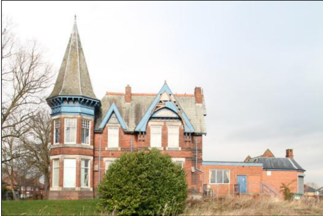
Plate 13: East elevation of Burnholme, looking northwest
