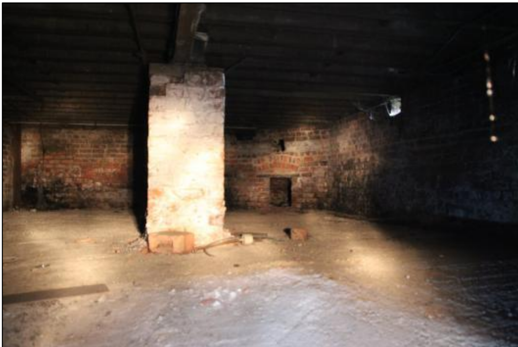
Plate 34: Room B4, looking southeast
