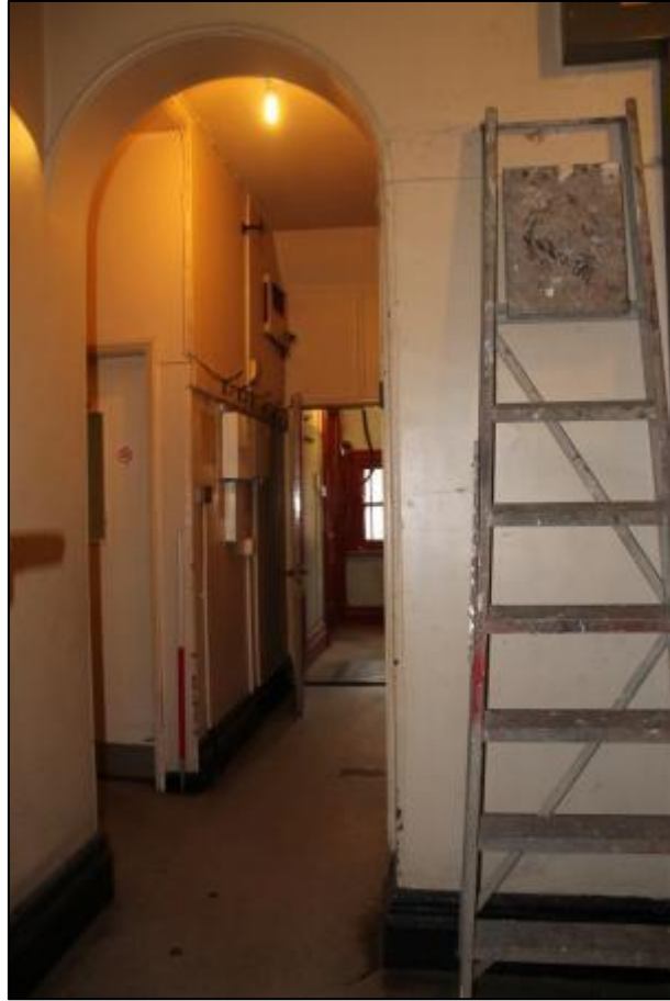
Plate 67: Room G6, looking northwest
