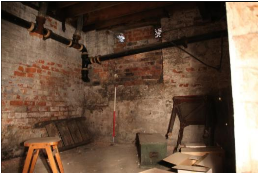
Plate 38: Room B11, looking west
