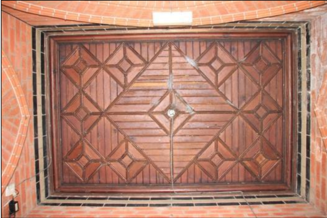
Plate 7: Panelled ceiling to porch
