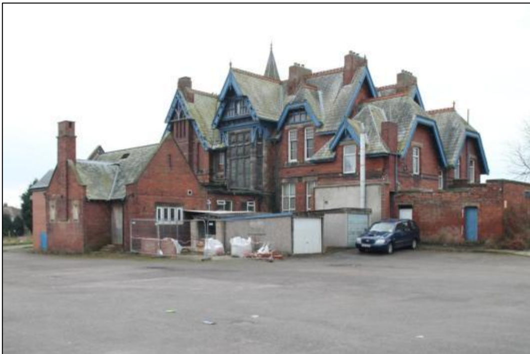
Plate 16: General view of northeast elevation
