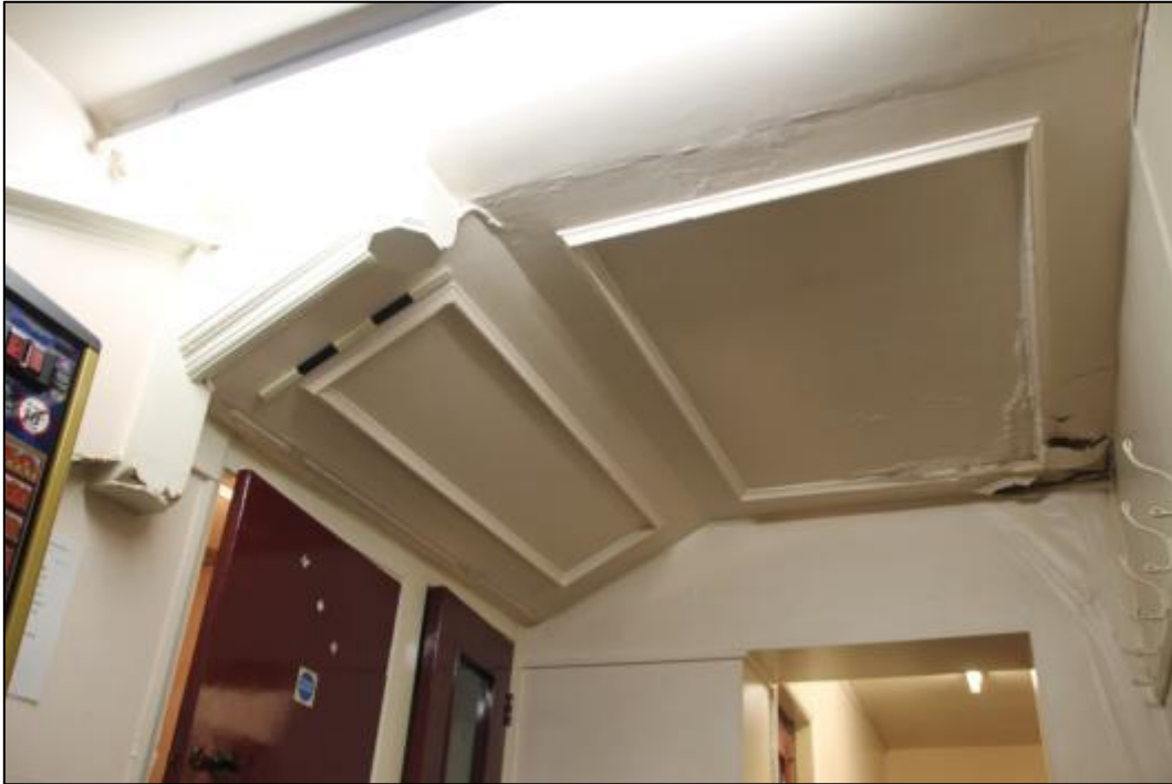
Plate 43: Detail of underside of staircase in Room G1, looking north
