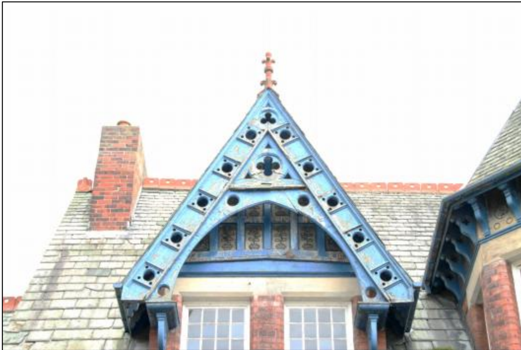
Plate 11: Gabled dormer above north bay of southwest elevation
