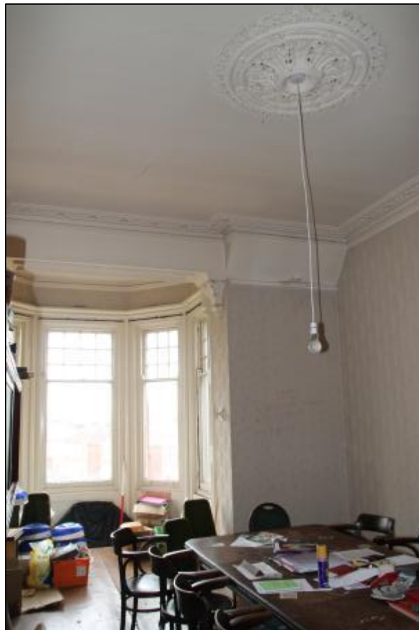
Plate 87: Room F4, looking southwest
