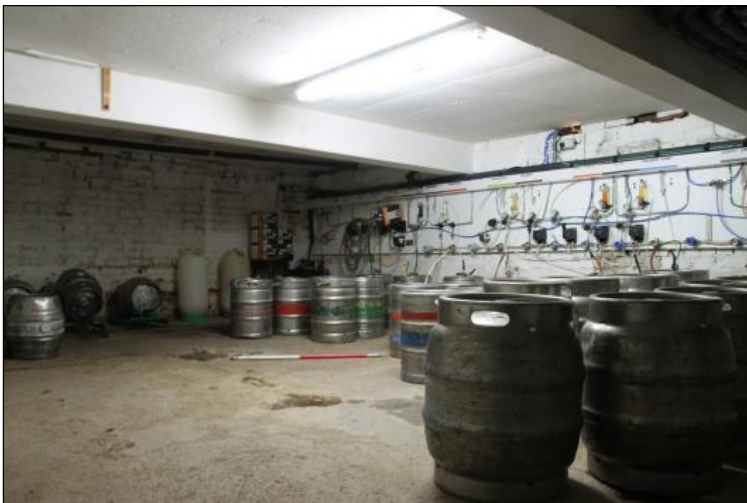
Plate 36: Room B7, looking west
