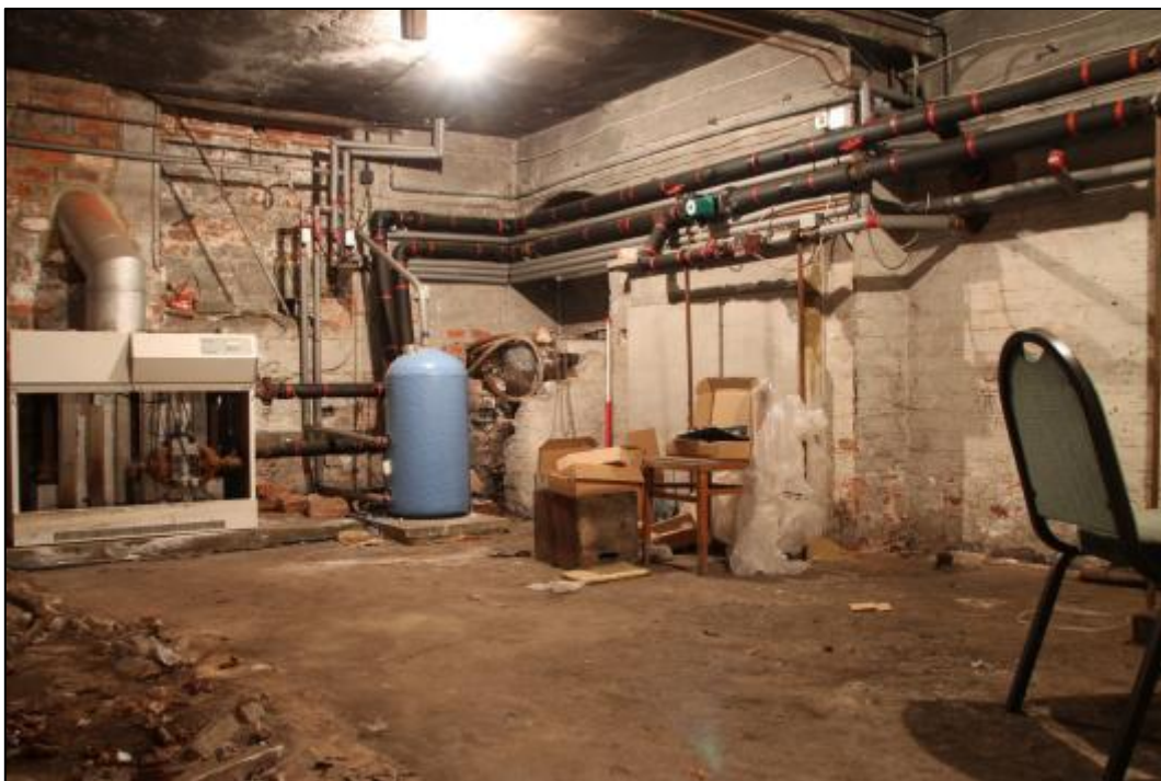
Plate 40: Room B13, looking east
