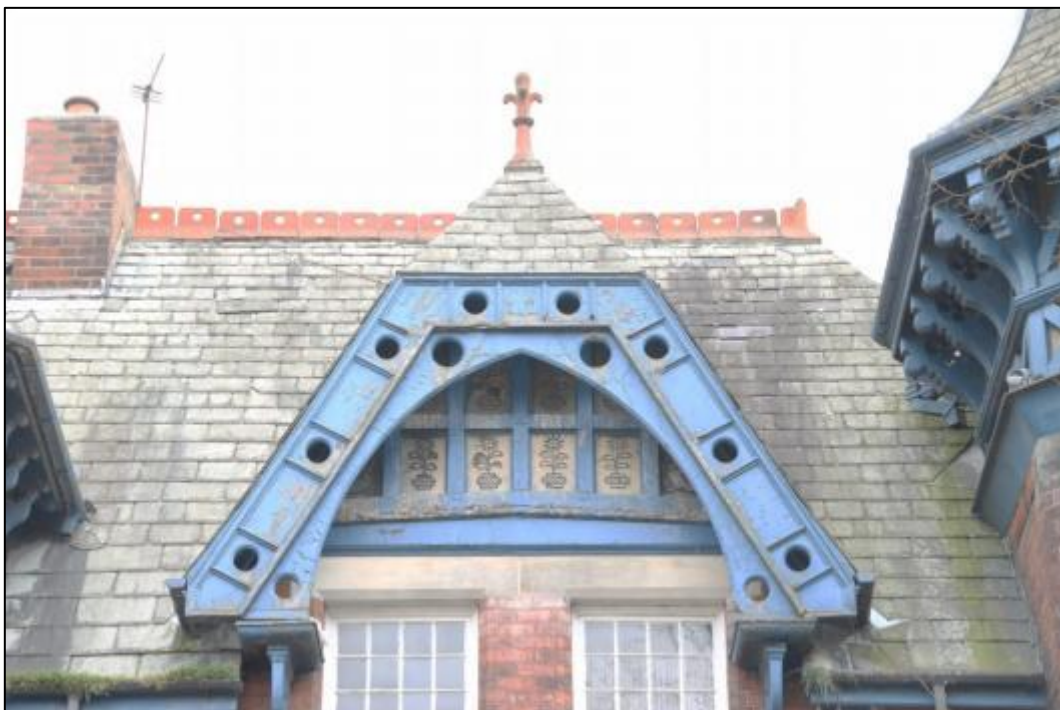
Plate 12: Gabled dormer above south bay of southwest elevation
