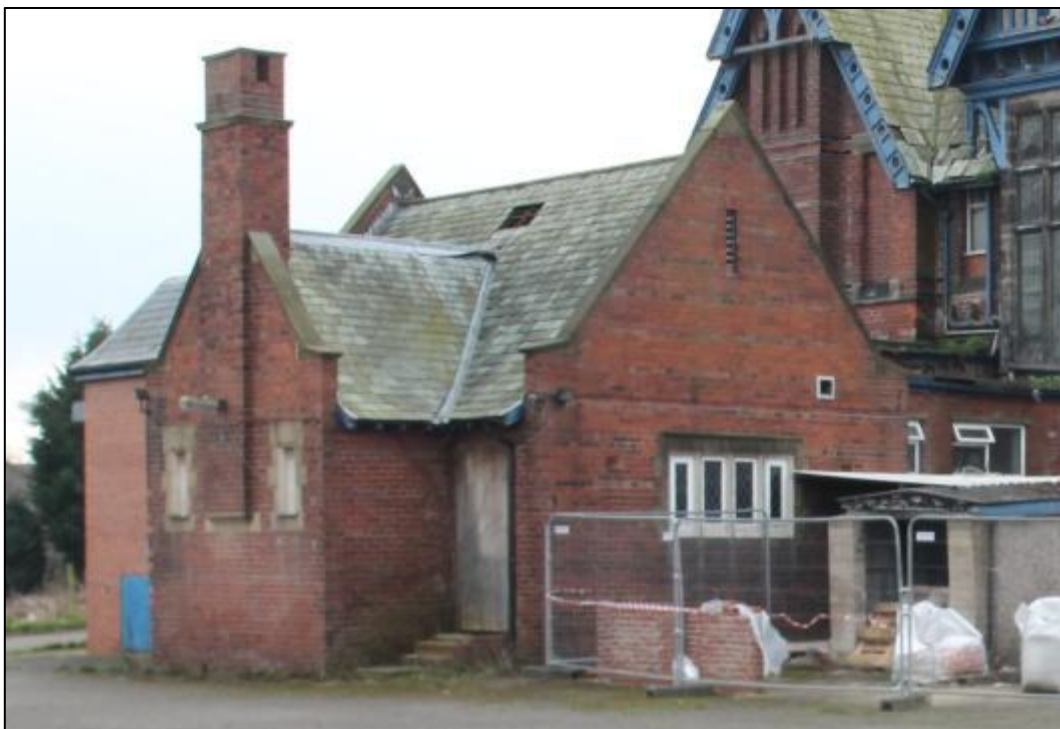
Plate 28: General view of pitched roof extension, looking south
