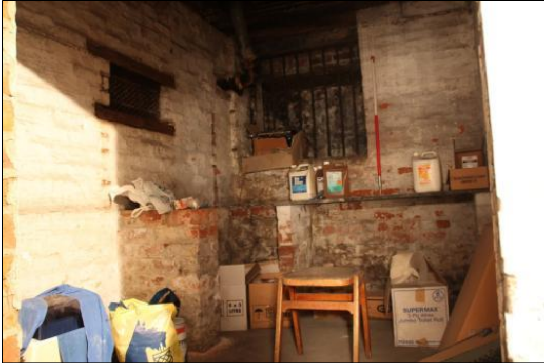
Plate 39: Room B12, looking west
