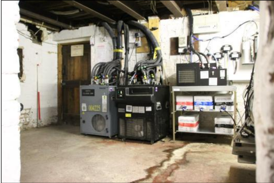
Plate 35: Room B6, looking east
