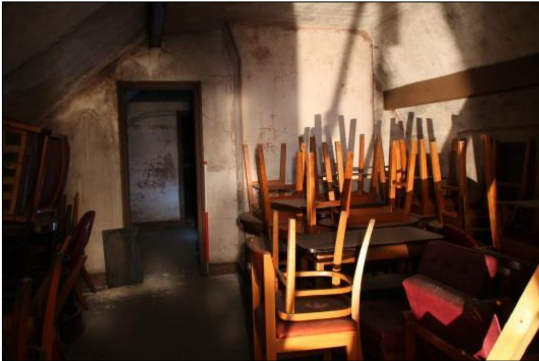
Plate 108: Room A6, looking southeast
