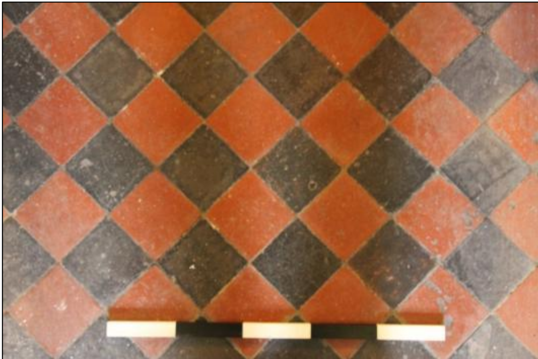
Plate 68: Detail of tiled floor at northwest end of Room G6
