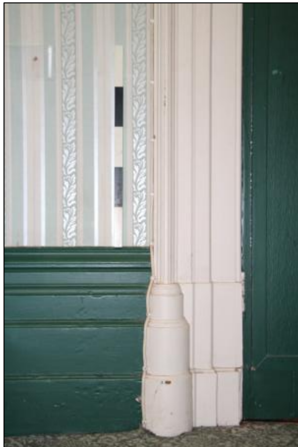
Plate 56: Detail of skirting and door architrave in Room G5, looking northeast
