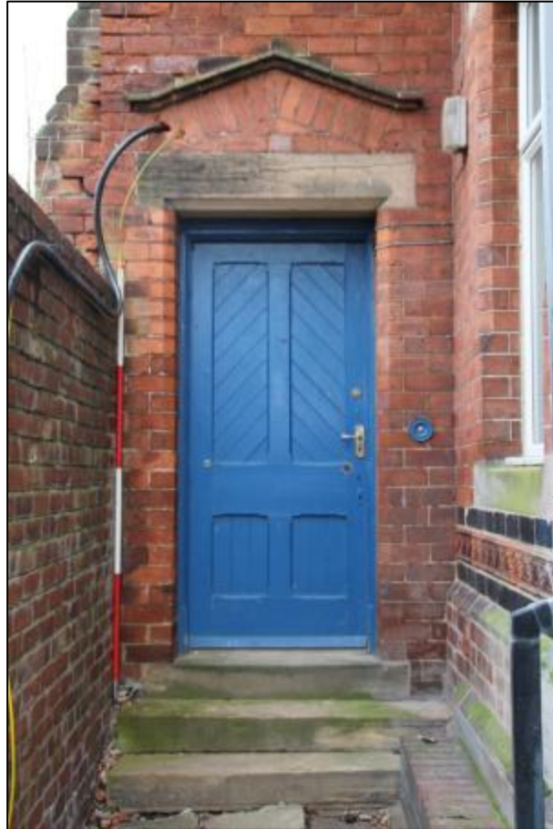
Plate 23: Former service entrance to Burnholme
