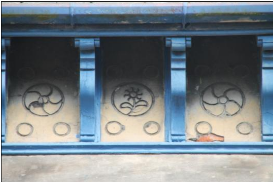
Plate 10: Decorative plaster panel above bay window at centre of southwest elevation
