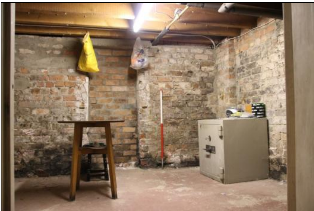
Plate 32: Room B3, looking southeast
