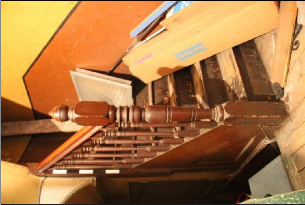
Plate 97: Room F7, looking north
