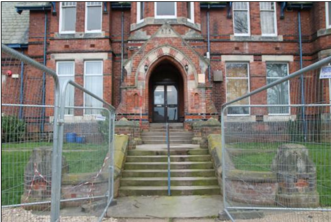
Plate 2: Porch on southwest elevation
