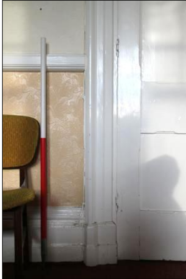
Plate 94: Room F5, detail of skirting and architrave
