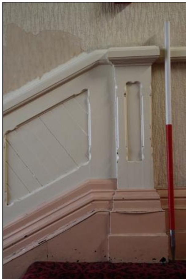
Plate 74: Detail of panelled dado on southeast side of stairs in Room F1
