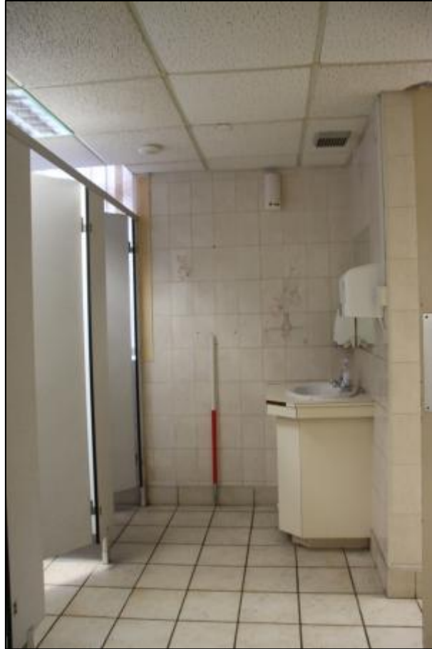
Plate 69: Room G9, looking northwest
