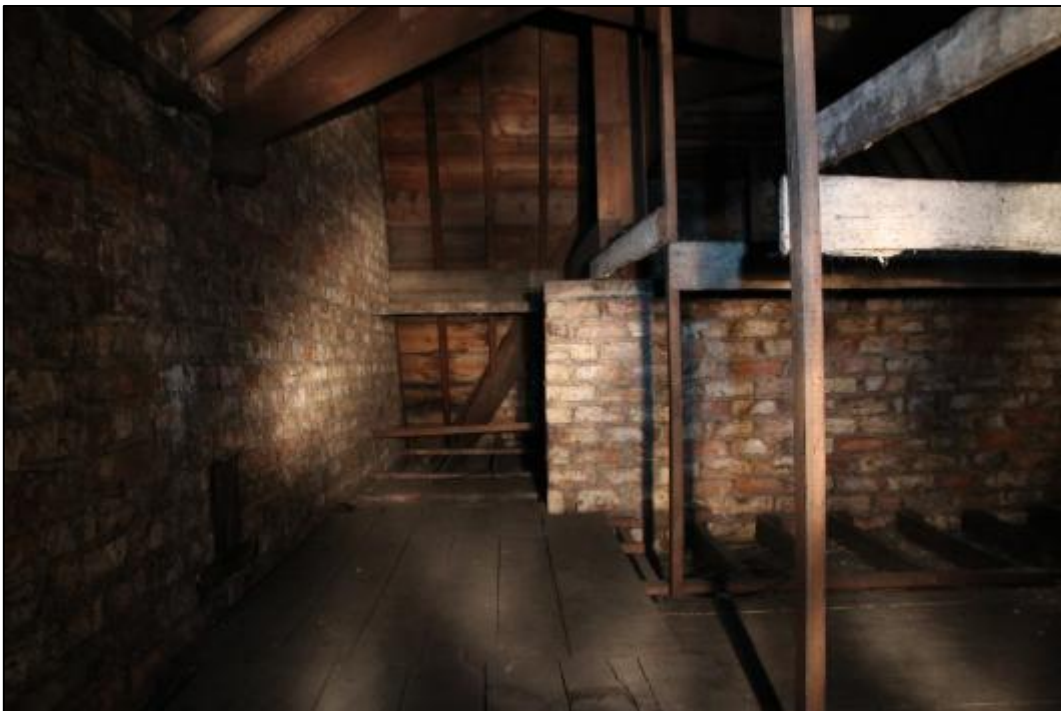
Plate 111: Room A9, looking northeast
