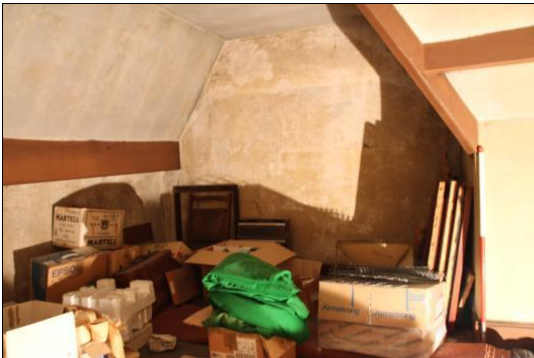
Plate 107: Room A5, looking west
