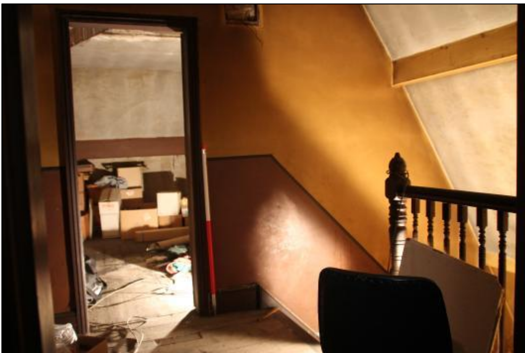
Plate 103: Room A1, looking west
