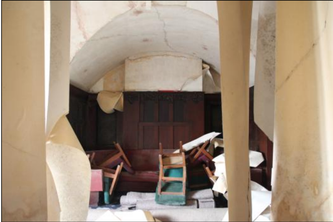
Plate 57: Room F7, looking northeast
