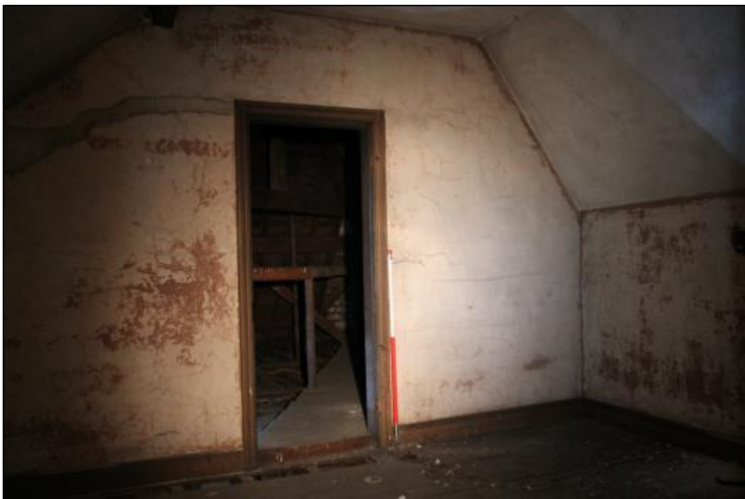
Plate 109: Room A7, looking southeast
