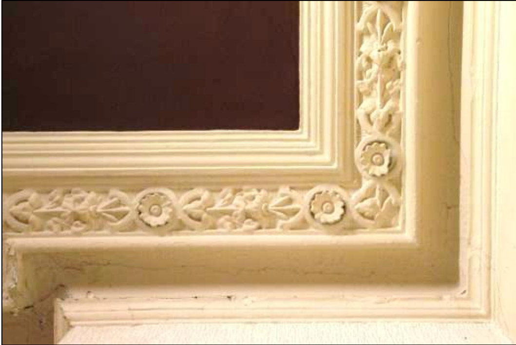
Plate 77: Detail of cornice in Room F1
