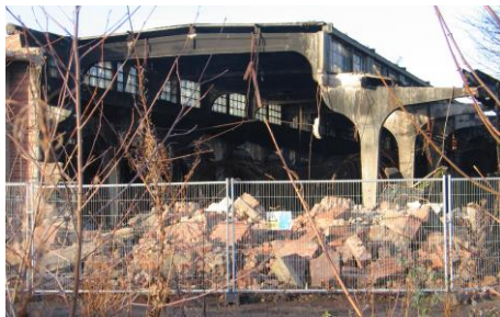
Store sheds of 1952 (Inventory no. 70) with a cantilevered concrete frame designed by John Dosser, demolished 2008
