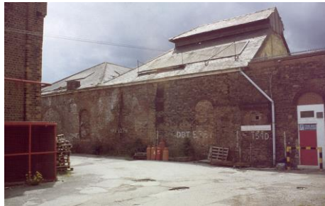
Phoenix Iron Foundry (Demolished)
