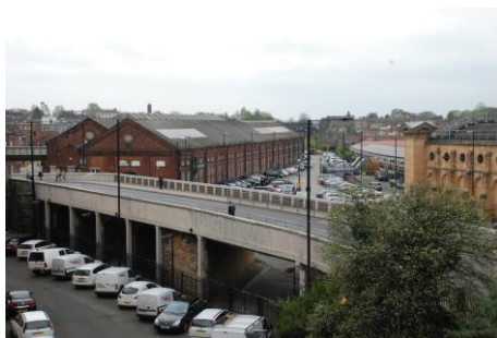
Queen Street Bridge
