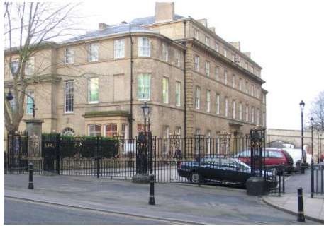
The First Royal Station Hotel of 1853
