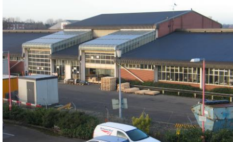
Signalling Maintenance Centre
