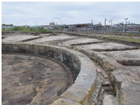
The excavated turntable and inspection pits
