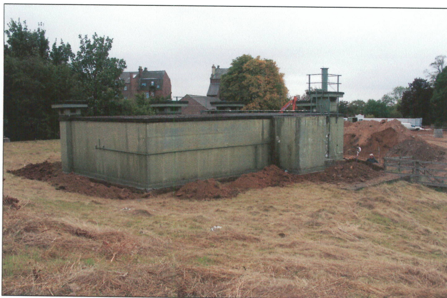
Plate 3: SE view of the rear of the main entrance structure
