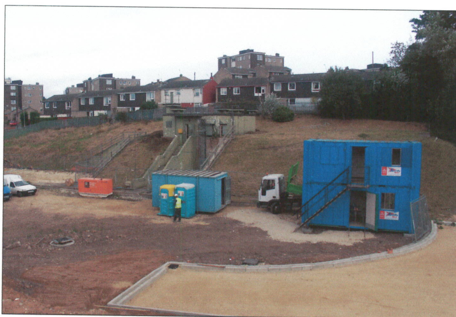
Plate 4: General view of the bunker looking north
