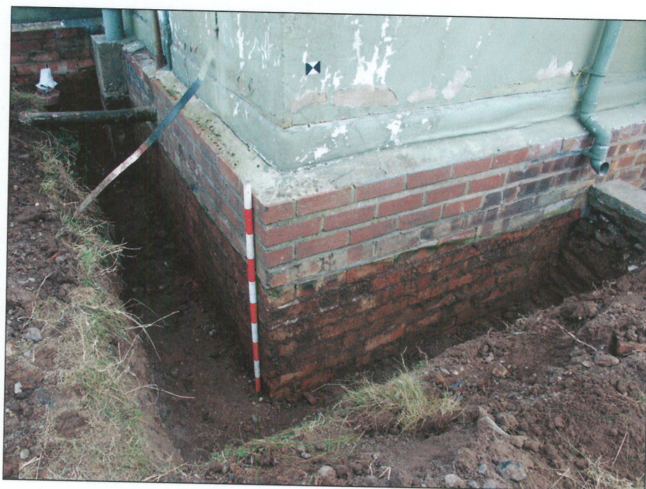
Plate 1: SW corner of main entrance block showing foundation trench
