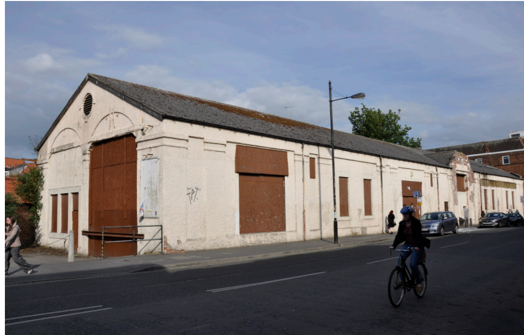
Former York Trolleybus Garage is vacant and at risk
