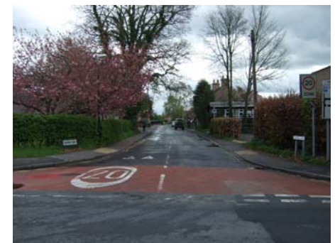
Plate 50 Excessive signage and road markings
